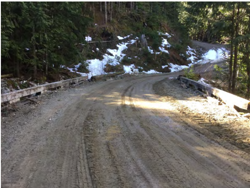
Approach from Right Bank when facing downstream
