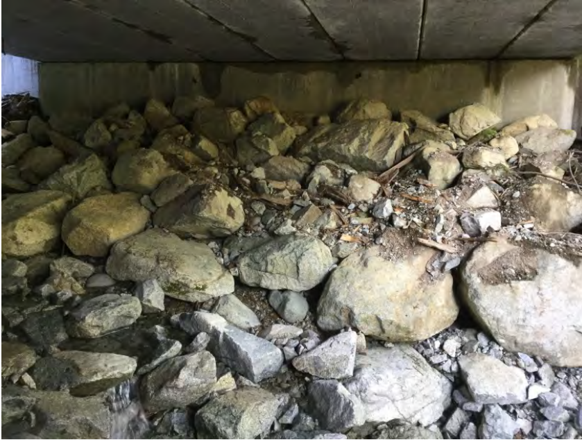
Left Bank Abutment when facing downstream
