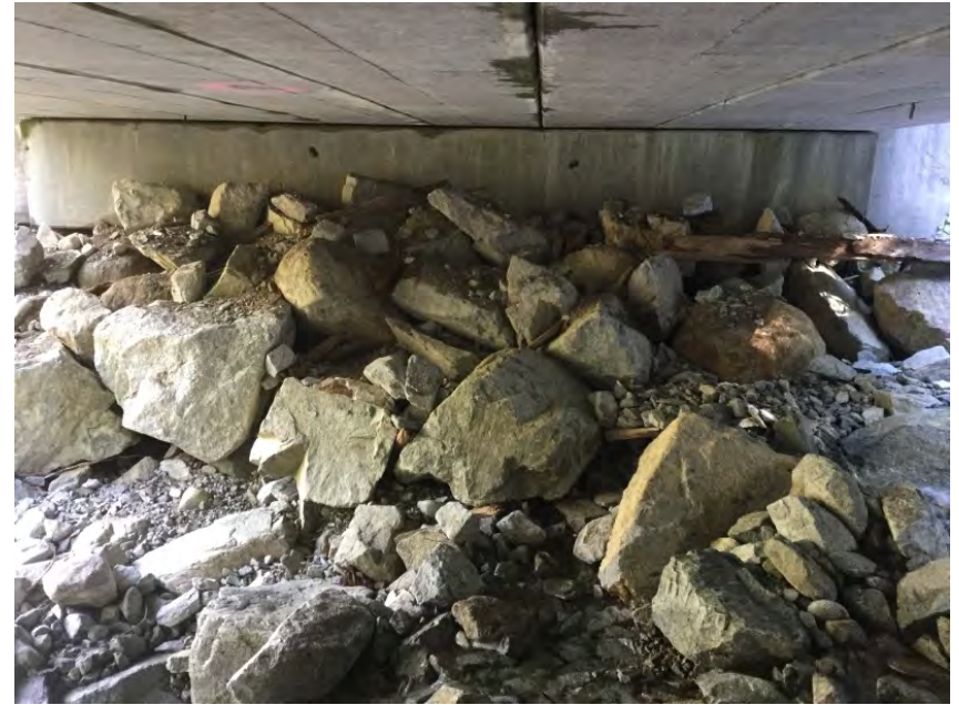
Right Bank Abutment when facing downstream
